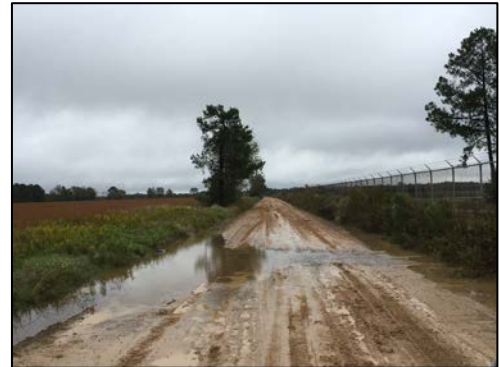
Photograph 2-1. Hightower Road from West to East with the Moody Air Force Base Boundary Fence Located to the South
